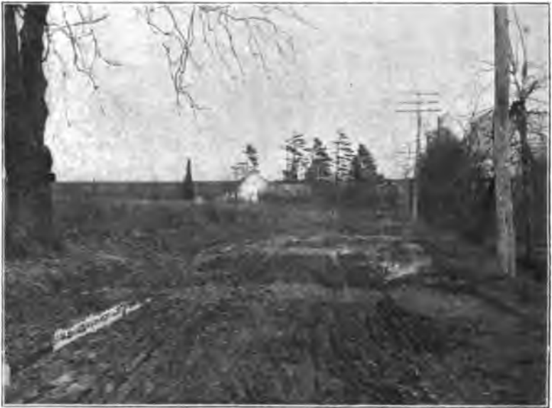
River road, near Phila. and Reading Railroad crossing, Mercer Co., before improvement.
